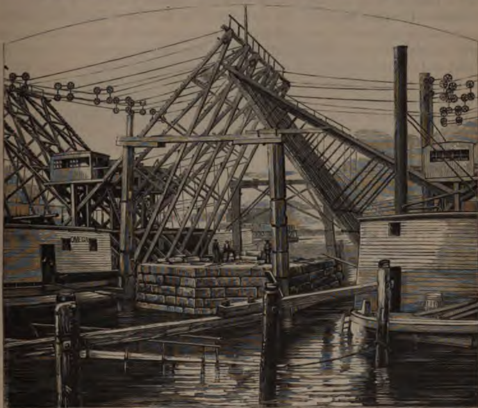
The building of the East Pier of the St. Louis Bridge.
